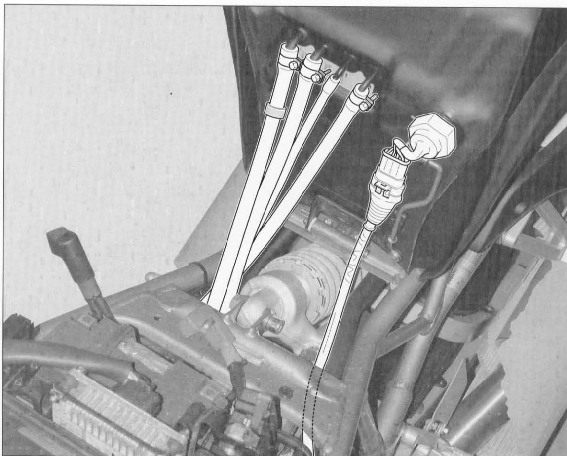
Arrangement of fuel level sensor tank hoses
